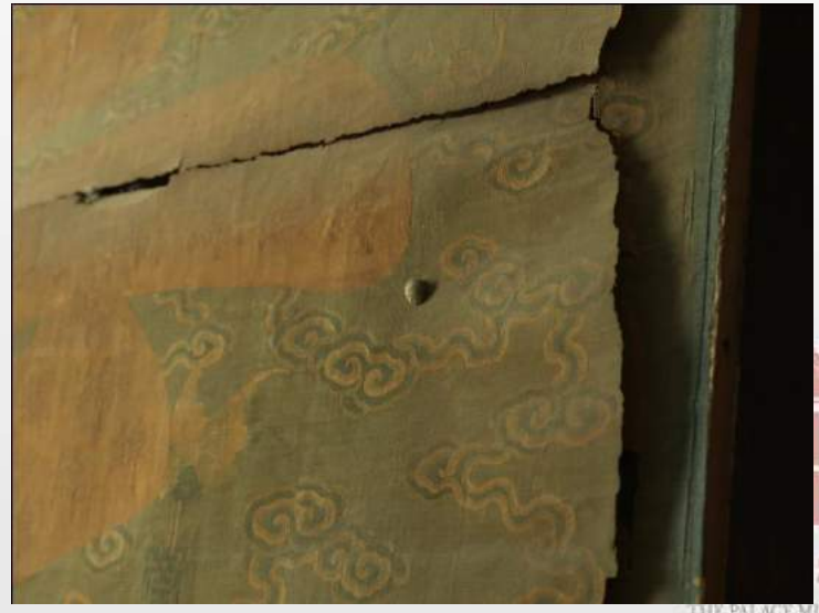
按钉的不良加固Wrong Consolidation
